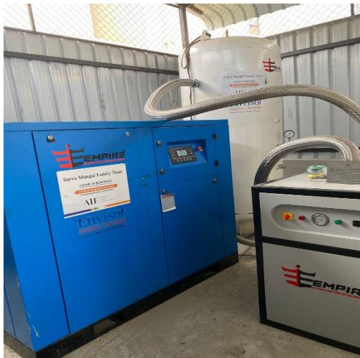
Oxygen Generation Plant
