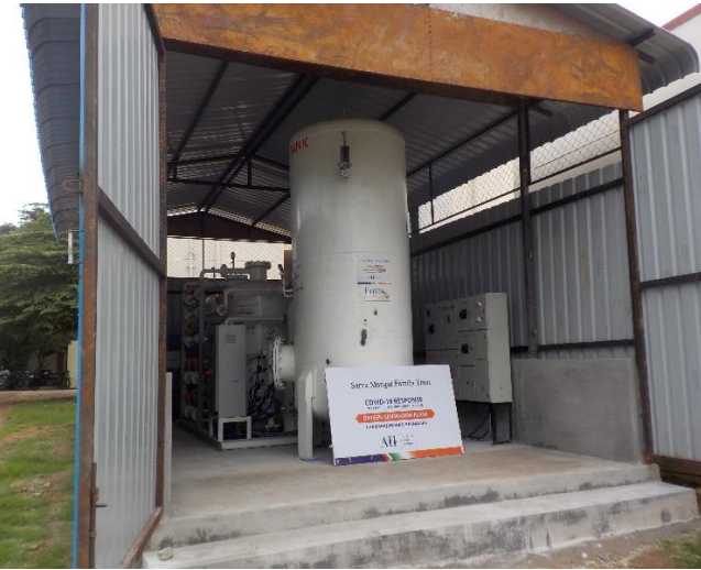
Oxygen Generation Plant
