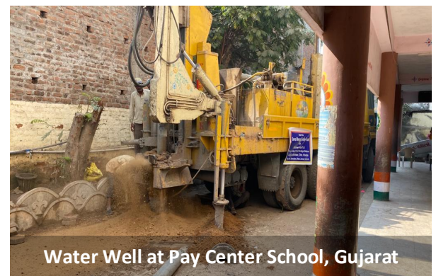
Water Well Digging
